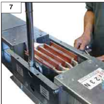
7 PERFORM THE TORQUE 60NM WITH DINAMOMETRIC TOOL
